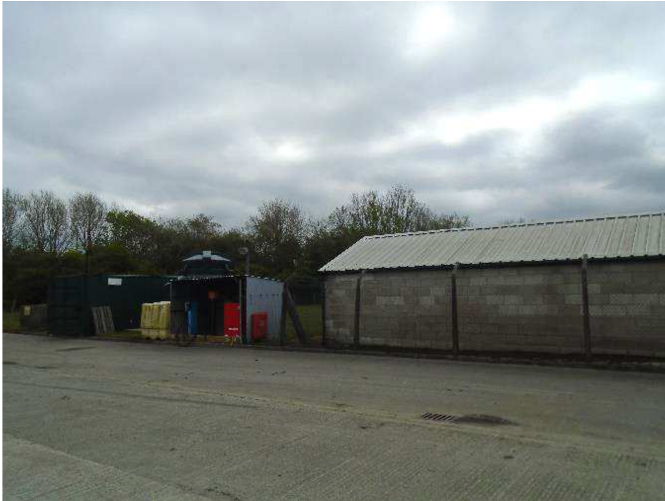
Location for the detention tank kiosk following removal of existing building
